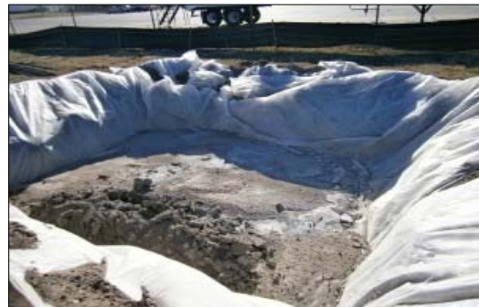
Plate 4-4 Concrete washout area
