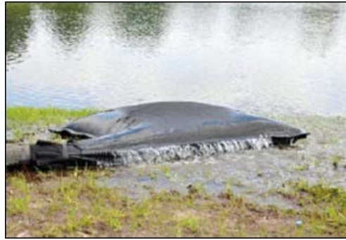
Plate 4-4 Silt bag under inspection
