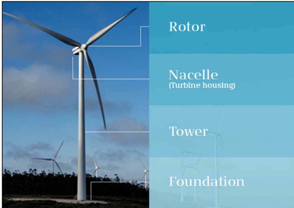
Plate 4-1 Wind turbine components
