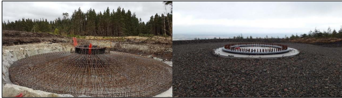
Plate 4-2 Turbine 'Anchor Cage' and finished turbine base
