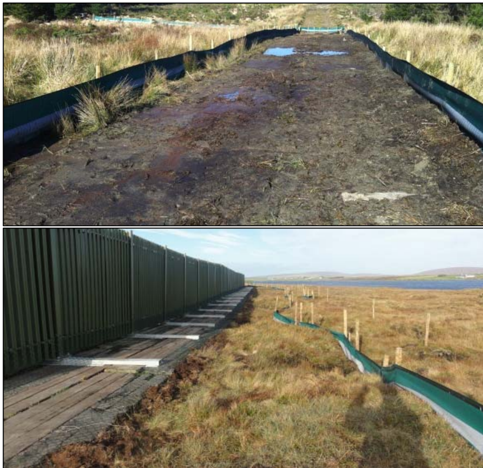
Plate 4-6 Silt Fence Details
