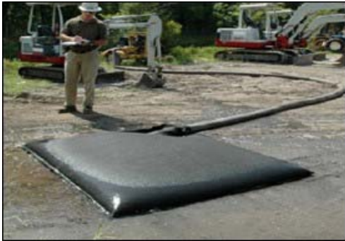
Plate 4-3 Silt Bag with water being pumped through
