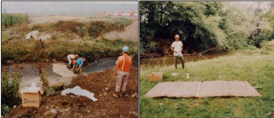
Plate 4-5 Typical Sedimat Details (Source: https://www.hy-tex.co.uk/ )
