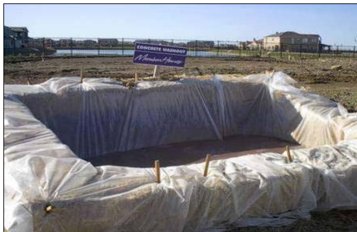
Plate 4-3 Concrete washout area
