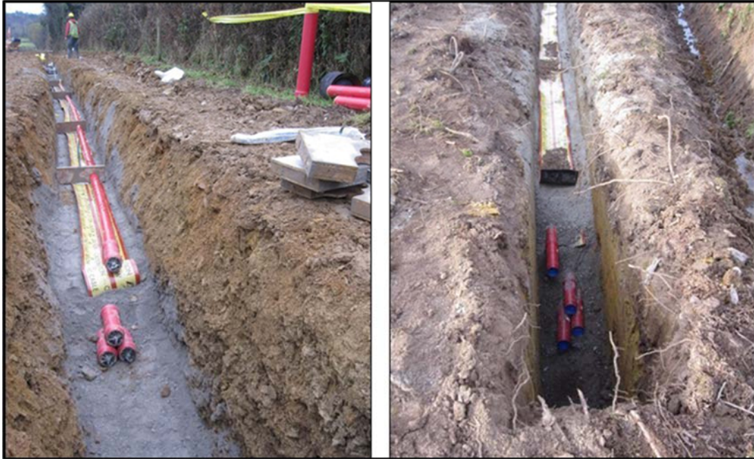
Plate 4-3 Standard Cable Trench View
